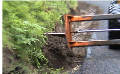
The Ditchpro Bucket can be extended to allow the removing of debris with the wheel loader remaining on the road surface
